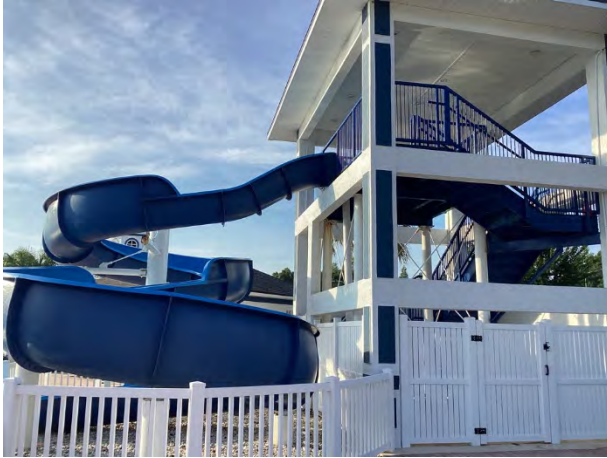
Water slide and staircase overview
