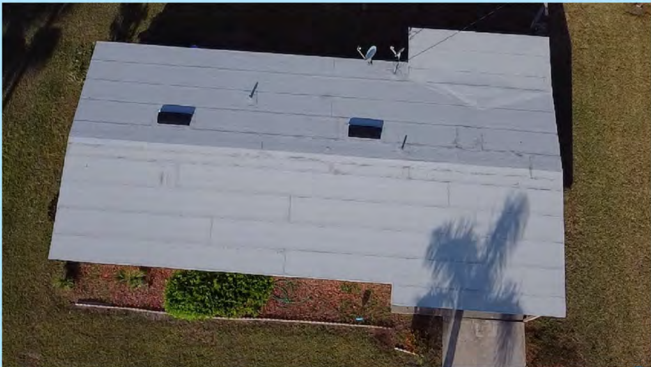
Modified Bitumen Roofing
